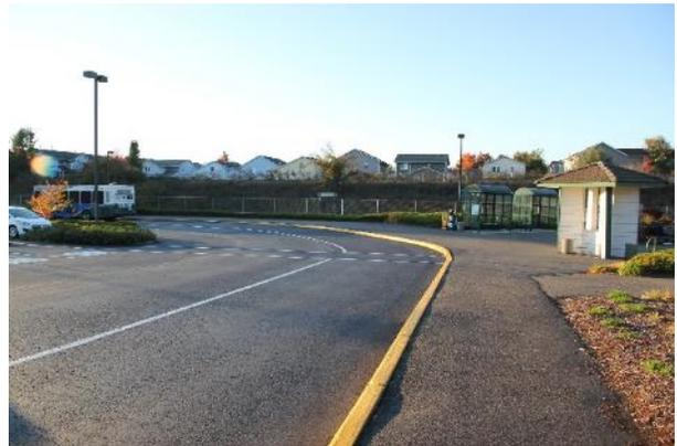
Photo 2: Yellow marked curb for bus routes with wide sidewalks.
