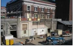
Above, the enclosure for the stairs and escalators to Jackson St. has been removed, along with the stairs and escalators. This was not a part of the original station. The open stairway build as part of the original building will be restored.
